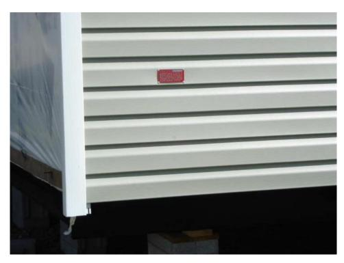
Look on **all bottom corners** of the home (left and right of each side). Double-wides and single-wides can be different with the location of the HUD Plate.
