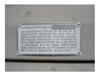
A HUD plate is 2<sup>nd</sup> best to the Data Plate and is still useful for acquiring the VIN. It does **not** have the VIN on it, but the HUD numbers will still help us get the VIN.
